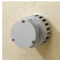
Balanced Flue (No chimney required) BF
